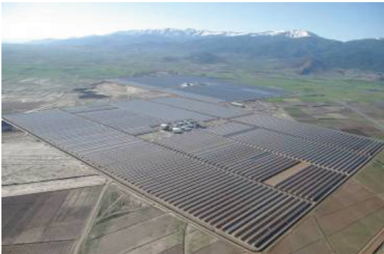
The ANDASOL 1 and 2 each generate 50 MW with 7.5 hours of storage (using molten salt), located in the province of Granada, Spain. Photo courtesy of Protermo Solar.
