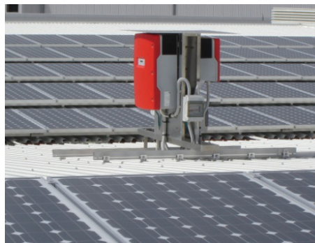
The Auckland Airport has a grid-connected PV Solar system. Photo courtesy of SEANZ.
