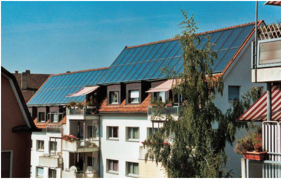
A solar hot water system is installed on a multifamily house in Zurich. Photo courtesy of Cobra.
