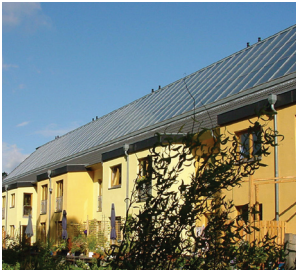
Roof-integrated flat plate collectors are shown. Photo courtesy of Wagner & Co/ESTIF.
