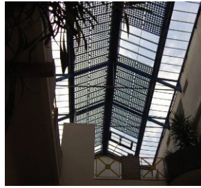
BIPV installation is shown. Photo courtesy of Enerplan.
