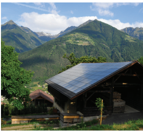
Solar panels on a barn in Southern Germany. Photo courtesy of Kyocera/Stromaufwärts.
