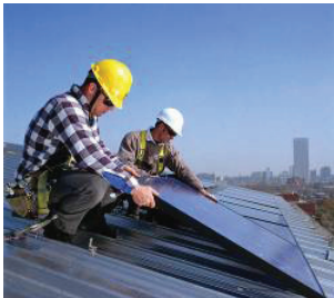
Workers install PV panels on a rooftop. Photo courtesy of DOE/NREL.
