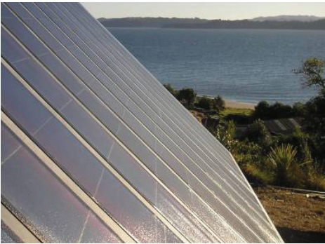
A PV Solar array provides Motuora Island with electric power. Photo courtesy of SEANZ.
