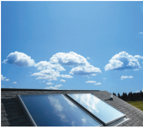
Solar PV panels collect the sunlight and produce electricity on a home in the U.S. Photo courtesy of Velux.
