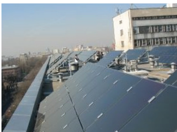
The outdoor test facility at Warsaw University of Technology. Photo courtesy of Polish Center for PV.
