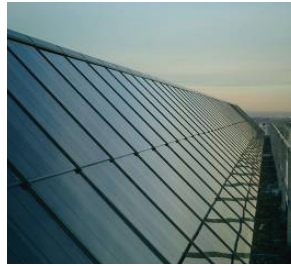
A large solar thermal installation is shown on the roof in France. Photo courtesy of Enerplan.
