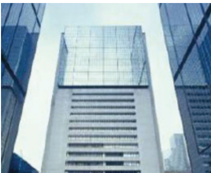
This photo shows the eco-friendly Suntech building—China's single largest building with integrated PV installation. Photo courtesy of SNEIA.
