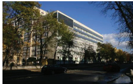
A 53.5 kWp system at the Warsaw University of Technology is installed on the façade. Photo courtesy of Center for Photovoltaics.
