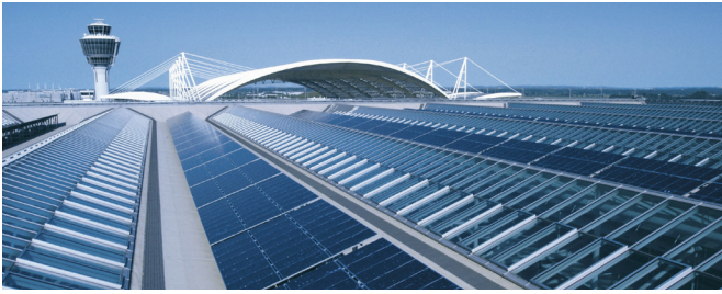
The Munich Airport has installed solar panels on many of its roofs. Photo courtesy of BP Solar.
