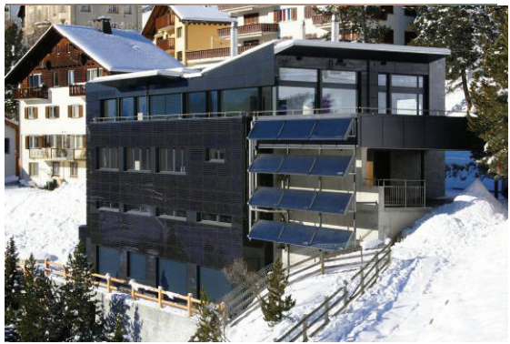
The façade of this house in St.Moritz displays a PV system. Photo courtesy of Swissolar.
