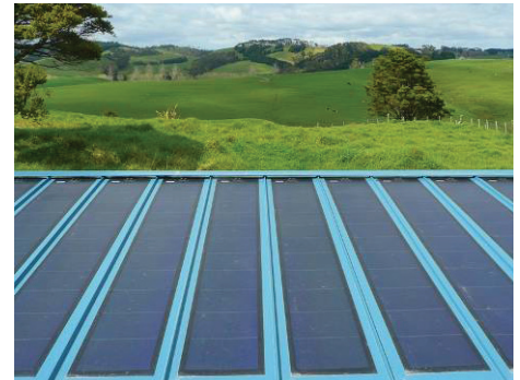
A grid-connected PV Solar array on the roof of a rural property is shown here. Photo courtesy of SEANZ.
