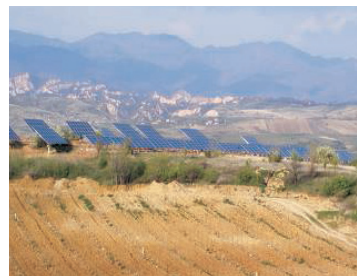
The first large PV installation for Bulgaria, located in Zornitza. Photo courtesy of www.pv-nms.net.
