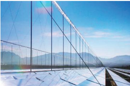
The Puerto Errado 1 is a Fresnel system with dry cooling that can generate 1.4MW. It is located in the province of Murcia, Spain. Photo courtesy of Protermo Solar.
