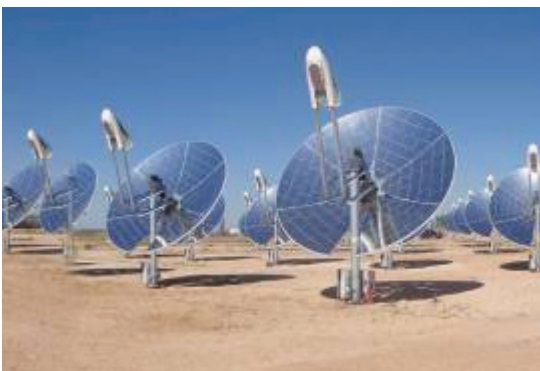
The Villarrobledo is a 1 MW Dish-Stirling plant in partial operation already in the province of Albacete, Spain. Photo courtesy of Protermo Solar.
