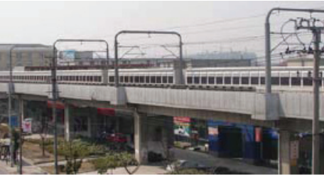
China's first thin-film cells also served as a sound barrier in an elevated rail bridge. Photo courtesy of SNEIA.
