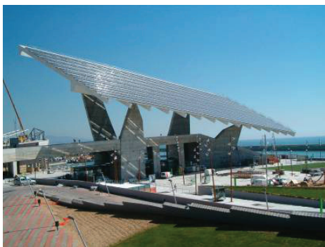
PV panels serve as the roof for this structure. Photo courtesy of ASIF.
