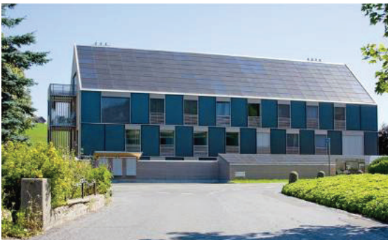
A multifamily “plus-energy”-house in Bennau has a PV installation on the roof and thermal collectors on the facade. Photo courtesy of Swissolar.
