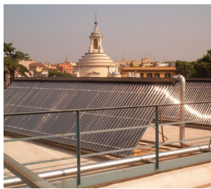
A hospital in Rome uses a solar thermal system with evacuated tubes. Photo courtesy of Thermomax/ESTIF.
