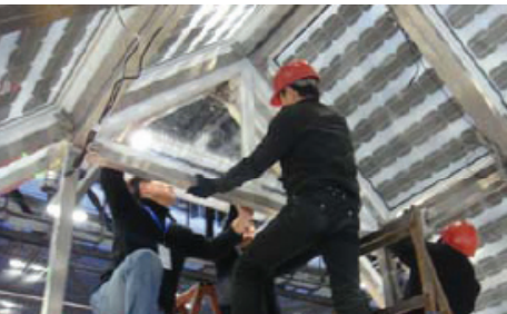
Workers install electricity generation equipment based on new embedded rooftop BIPV technology. Photo courtesy of SNEIA.
