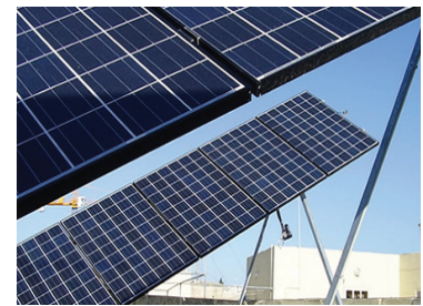
Rooftop solar panels are shown here in Malta. Photo courtesy of www.pv-nms.net.
